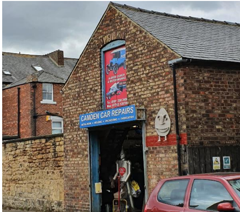
Former stable, Camden Place
