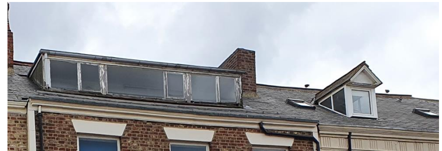
An unsympathetic boxy dormer on the left. The dormer on the right is more appropriate but is joined by rooflights that although small, disrupt the roofline
