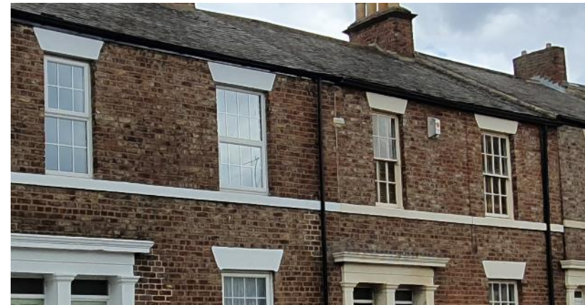
PVCu windows with flat, flimsy glazing bars and chunky frames, left, compared to traditional timber windows on the right
