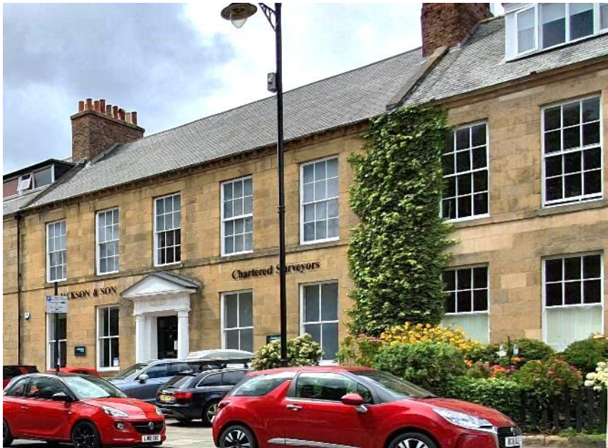
Vertical window openings, Northumberland Square
