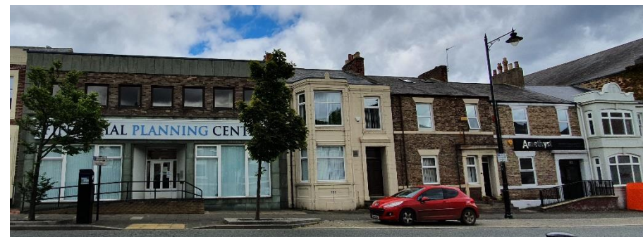
Complete loss of front gardens, Howard Street
