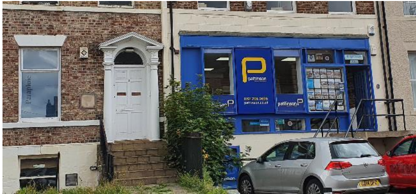
Inserted shopfront that does not respect the architecture of the building, Northumberland Place
