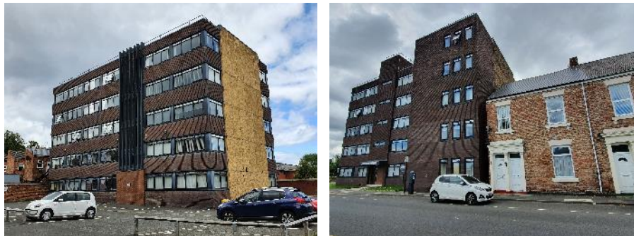
Stephenson House and car park, left, and its uncompromising scale, right
