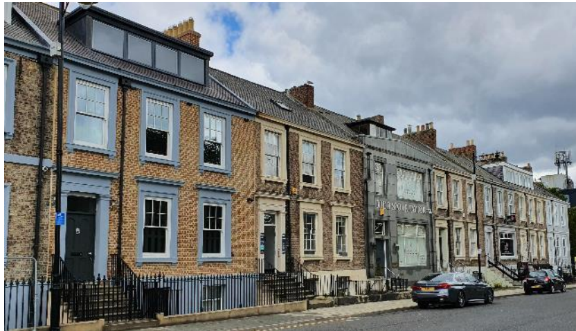
Painted sandstone sees the loss of the rich, natural material and harms unity
