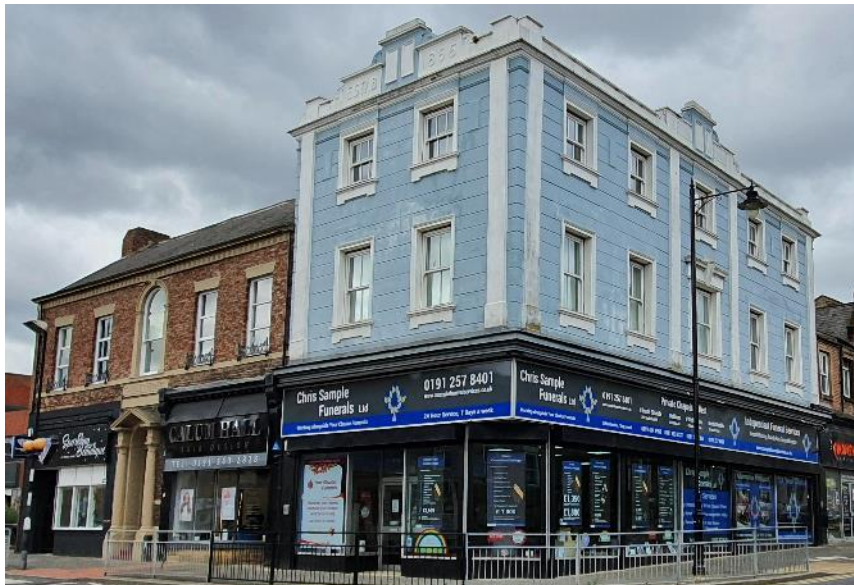
Modern shopfronts with large windows and fascias that harm the buildings' appearance
